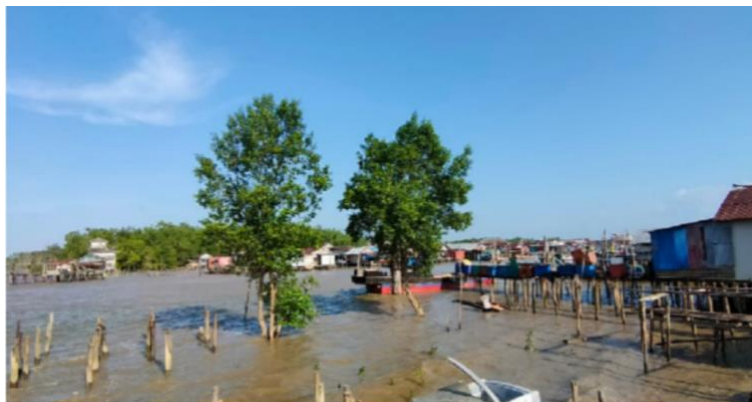
Figure 1. Condition of mangroves and coastal residential areas
