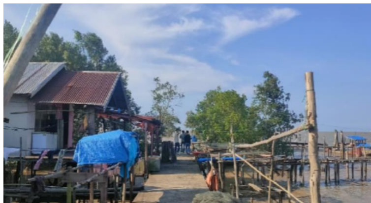
Figure 2. Condition of residential areas in coastal area
